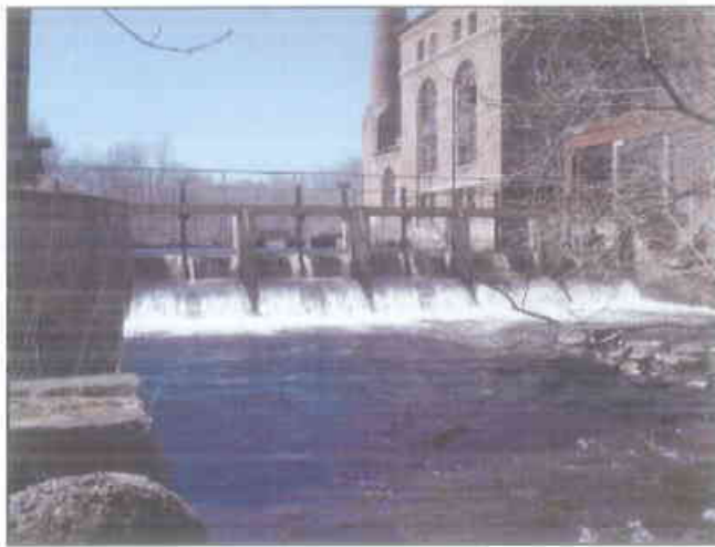
View of Baker Dam looking upstream.
