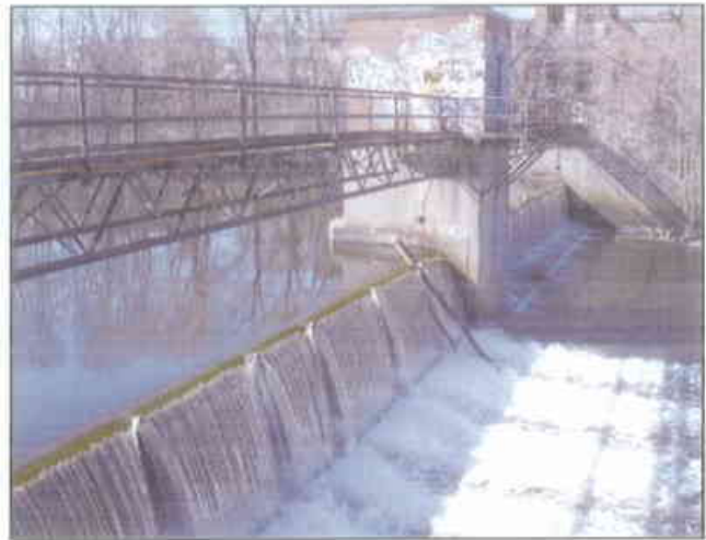
View of T&H Dam from the right bank.
