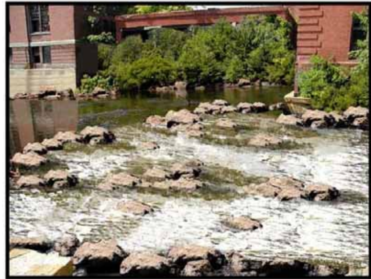
Photo-Simulation Partial & Complete Spillway Removal (Conceptual Fish Passage Shown)
