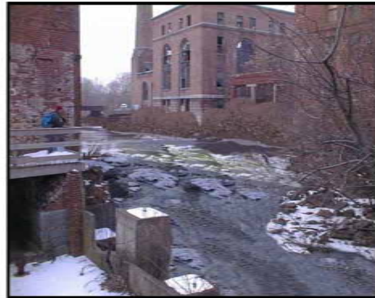
Photo-Simulation Partial Dam Removal with Rock Ramp (Conceptual Fish Passage Shown)
