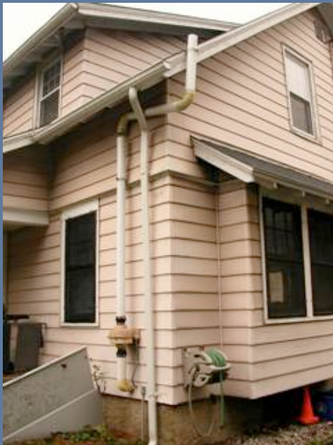
View of a home with a traditional Radon System
