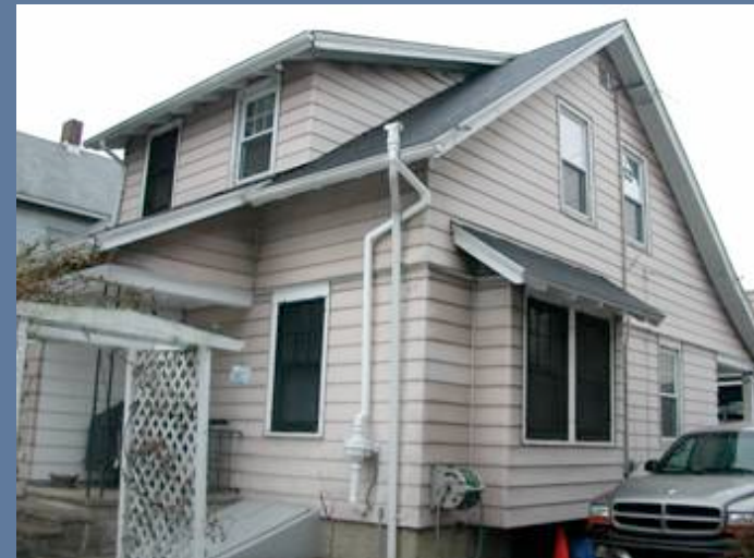
View of the home with the Engineered SSD System
